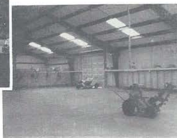
Interior of Golf Cart Storage Building. Capacity 50 Carts
