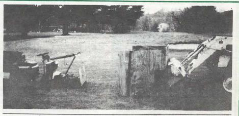
Apparatus invented by Ellis to cover his greens includes 4'x8' bucket and plow with brush attached to bottom ... #4 green in background covered with salt marsh hay and pine needles.
