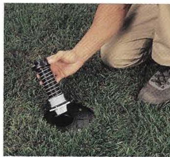
Then pull out heavy-duty snap ring with wiper seal to access gear-drive assembly.
