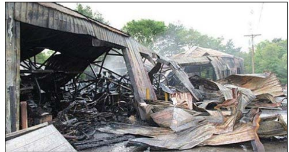
Photos courtesy North Reading Police Dept.
