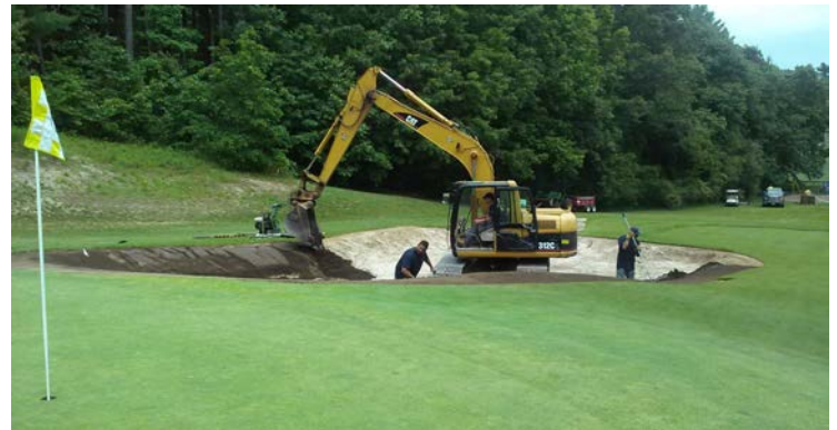
DHT Golf Services reconstructing a bunker at GCSANE field day
