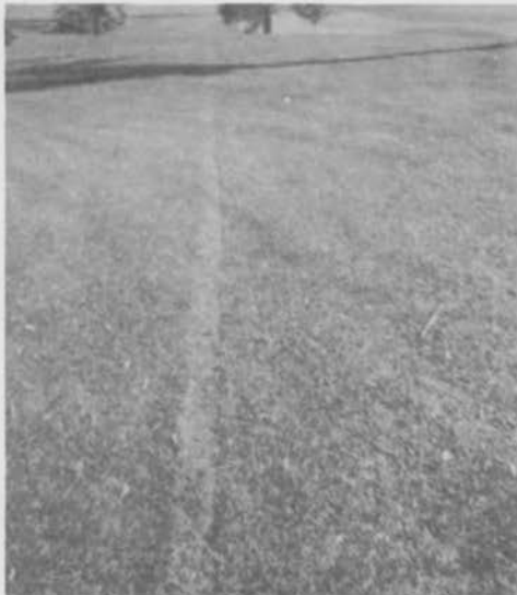
Sod replaced over wire. Out of danger from golf spikes and a tripping hazard removed from the gallery.
