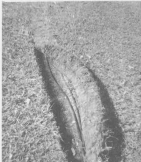
Slit made by sod cutter with wires placed in furrow and covered by sod. This is best done in damp soil for quick healing.
