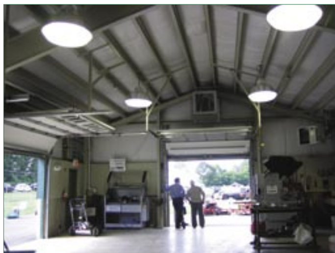
Shop/Equipment Storage Area.
