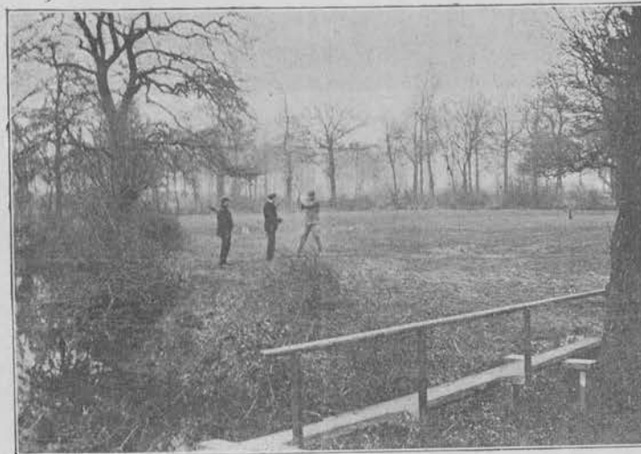
ONE OF THE GOLF BRIDGES.
