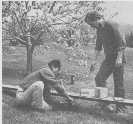
Jeff, U.M.C.C. Assistant Superintendent, and Cesar start construction of the main scoreboard.
