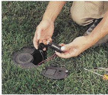
Remove solenoid, wire connections, pilot valve and adjustable regulator...
