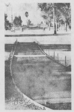
We have found that with our soil here in Mesa there is little or no need for an ABC base or additional compaction. Expansion joints are placed every 30' unless we pass close to a tree. This may vary for each course depending upon their local soil types and temperature extremes.
