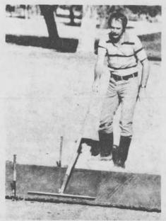
Because of the combination of foot traffic as well as cart traffic on grades varying from flat to steep and conditions varying from dry to wet, we have found that a very coarse to rough finish is necessary. The finished edge is accomplished with a rounded 4" edger.
