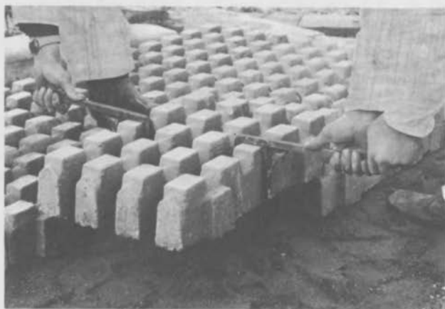
MONOSlabs permit lush grass to grow despite wear from wheels or feet.
