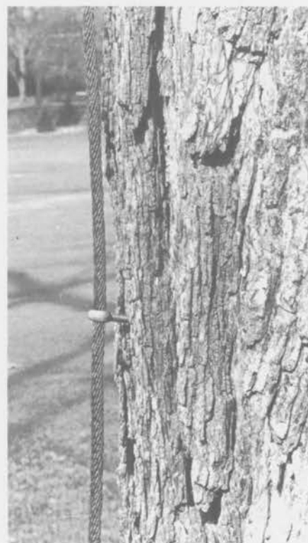
Copper cable connected to tree trunk
