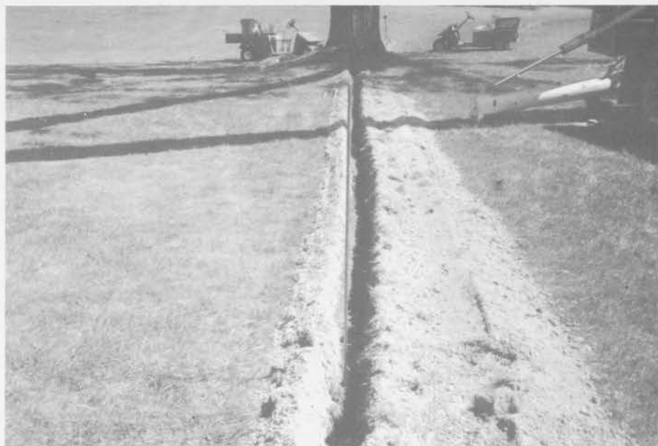
The trench is dug to the dripline so the cable can be placed in the ground and then connected to the grounding rod.
