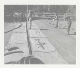
Laser level confirms trench grade; sod tamping begins.
