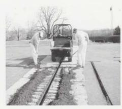
Four-wheeled carts remove excavated material.
