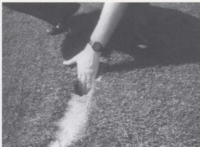
A 3-inch-wide slit drain just after installation.
