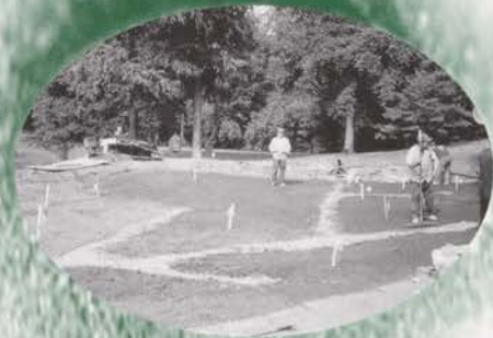
Drainage is installed with pea gravel, which is even with the subgrade.
