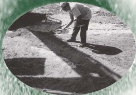
The 5-4-1 mix is coned over the drain lines.
