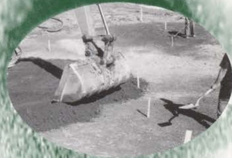
Soil is replaced just as it was taken out, using two, 4-inch lifts.
