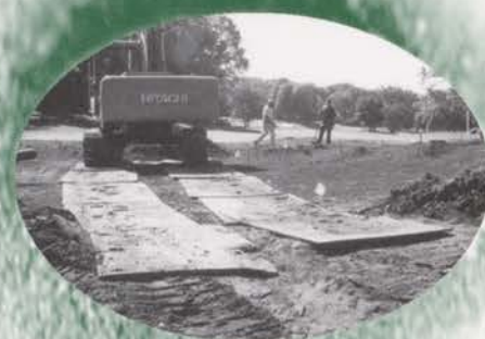
The subgrade is completed and the drain line cutting begins.
