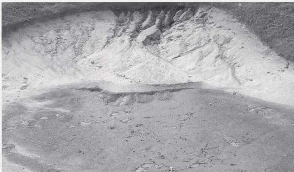
Poor drainage means the bunker will suffer from rapid contamination and will end up with a short life span.
