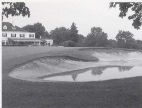
Bunker washout before rebuilding.
