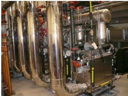
Heating system under BMO Field.
