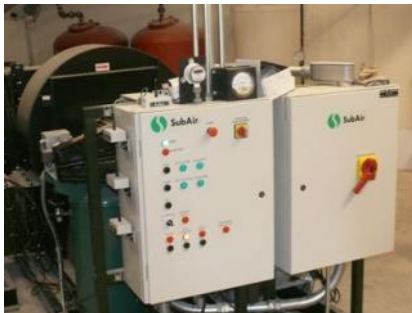
SubAir System controlling air and moisture of turfgrass on BMO Field.
