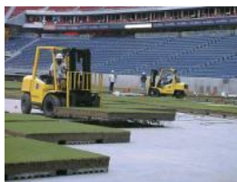
StrathAyr's Removable Natural Turf Surface being installed.
