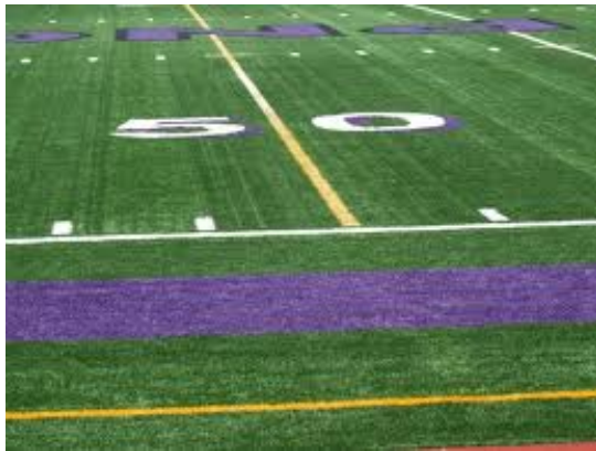
The artificial turf in Indian Stadium at Port Neches-Groves High School is showing premature wear.
