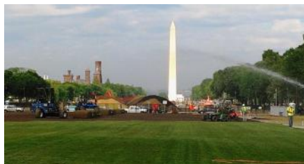
Newly laid sod being irrigated following installation.
