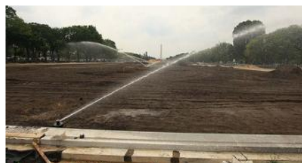
Testing of irrigation system prior to sod installation.
