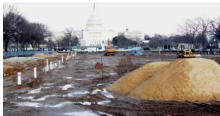
Irrigation pump station and the sub-drains installation.
