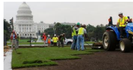
Installation of turf on engineered topsoil sand blend.
