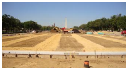
Coarse sand base awaits 6 to 18 inches of topsoil.
