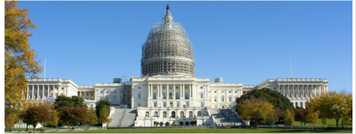
U.S. Capital under renovation. Photo by D. Ramey Logan
